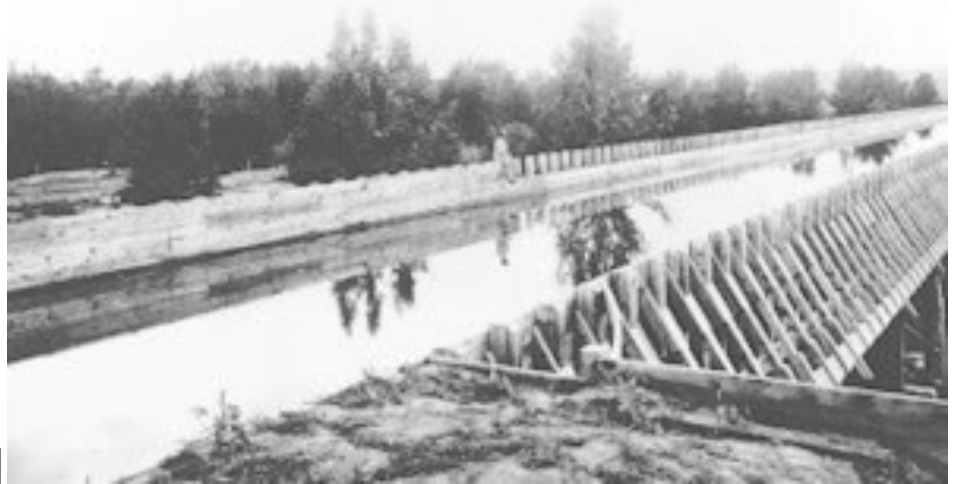
Highline Canal flume under construction in 1884 —Photo courtesy of Littleton Historical Museum
