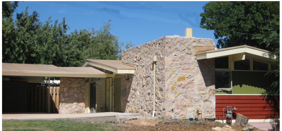
Many of the homes in the Arapaho Hills subdivision feature rhyolite rock walls and low-pitched roofs.
